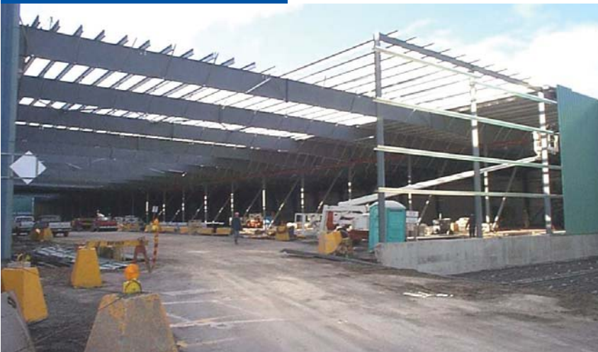
Phase 2 warehouse under construction
