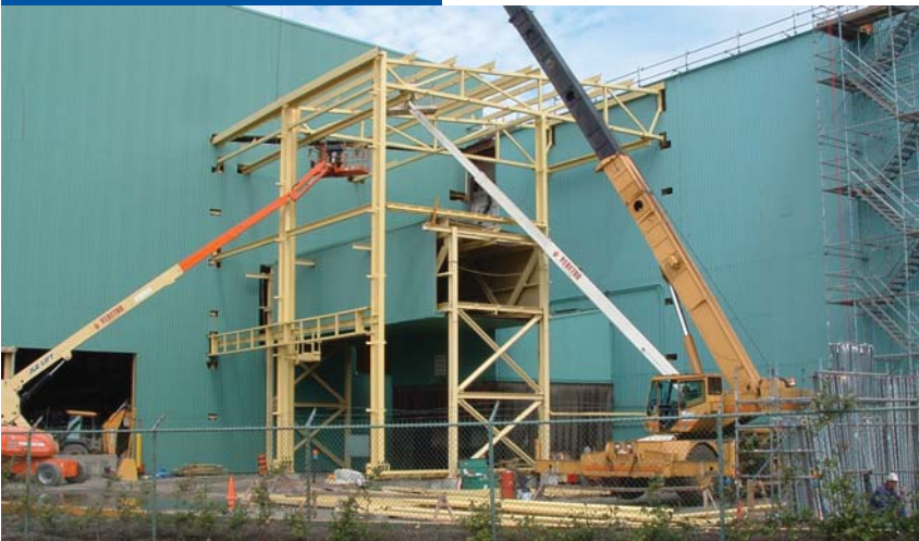
No. 2 CPCM Site – Erecting Side Trim Scrap Handling Building
